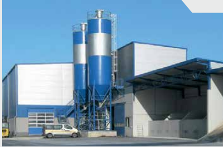
Concrete batching plant
